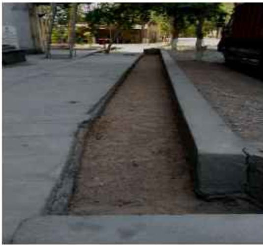
Rainwater harvesting recharge trench near bag house and near cement mill 2 area
