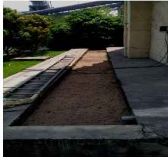
Rainwater harvesting recharge trench near bag house and near cement mill 2 area
