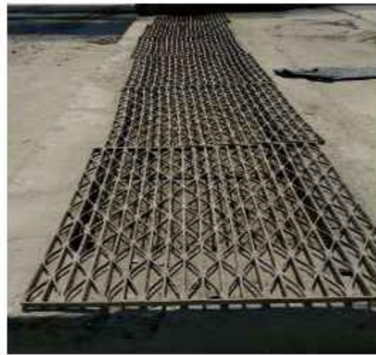
Rainwater harvesting recharge trench near bag house and near cement mill 2 area
