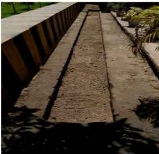
Rainwater harvesting recharge trench near bag house and near cement mill 2 area
